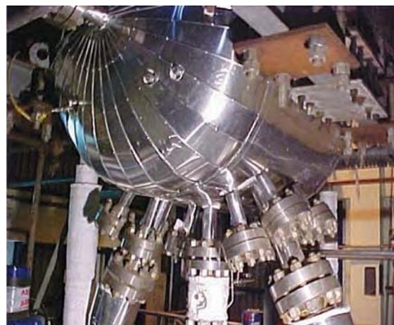
Fig. 12(b): Installed steam drum with tailpipe & downcomer connections for IFL
