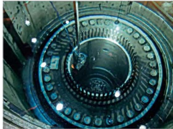
Fig. 15: WIM performing weld cleaning
