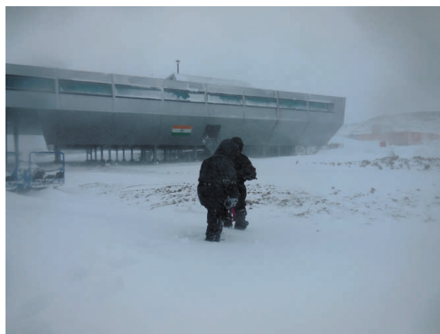
Fig.20: Snow drift in front of Bharati station
