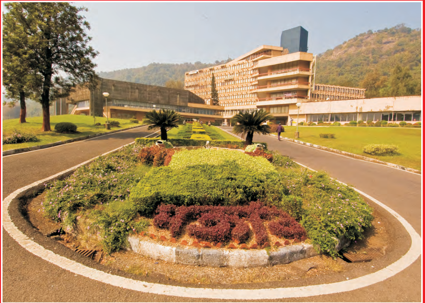
Central Complex BARC
