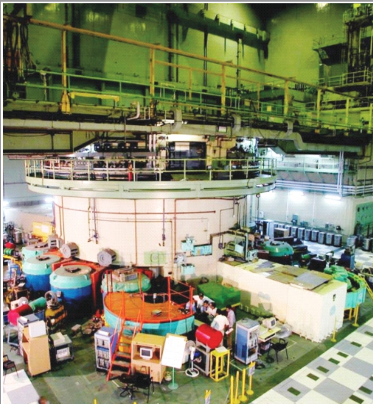
Dhruva Research Reactor Facility (Inside view)
