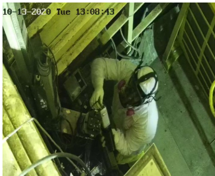
Camera replacement underway in maintenance area
