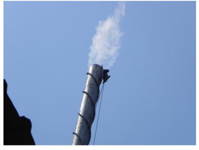
Primary Chamber Gaseous emission at 30 m Height Chemical Incinerator Plant : For disposal of legacy based organic chemicals and used Oils.
