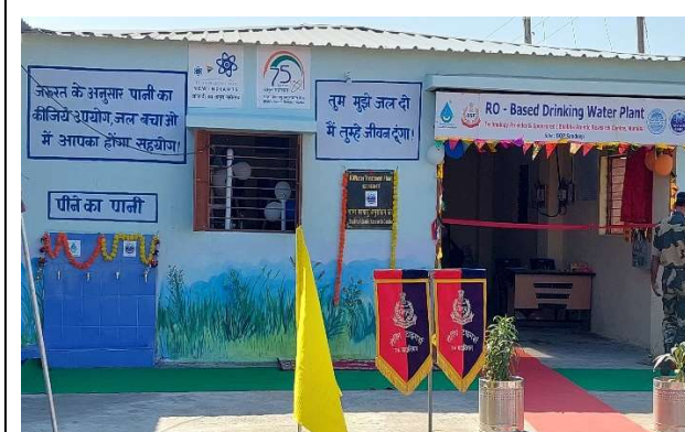
12500 LPH capacity water treatment unit
