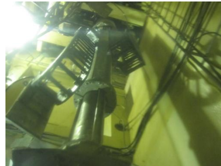
Vertical Cable Take-up for ASM inside Hot cell
