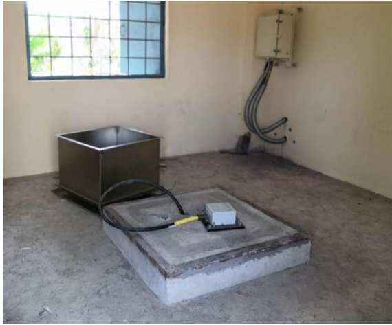
Indigenous Seismic Switch installed at KAPPS 3&4
