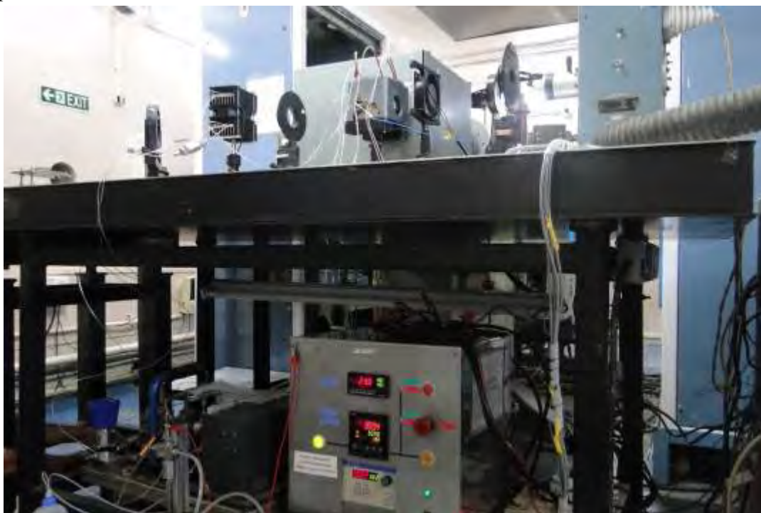
Fig. 2: High temperature high pressure set up installed at LINAC facility (bottom: control panel with pressure, temperature and flow display; top: optical cell inserted with four heating cartridges)
