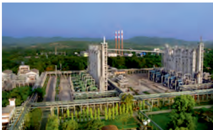
Heavy Water Plant, Manuguru
