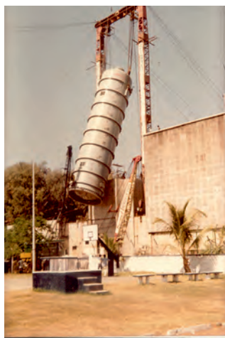
Fig. 4 (i): Installation stages of Pelletron
