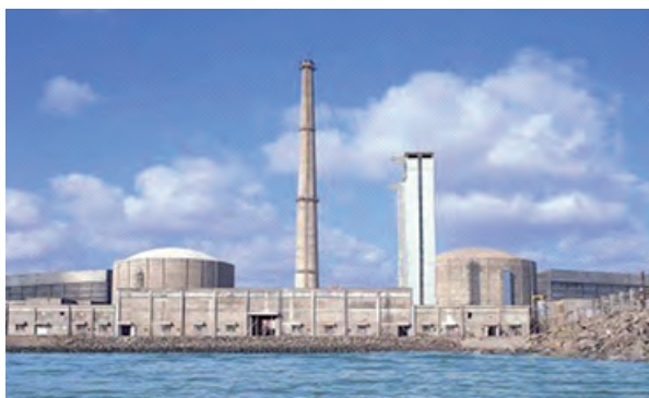
Fig. 3(a): 540 MWe Tarapur PHWRs Unit # 3 and 4. Nuclear plants do not release any pollutants and its carbon foot print is negligible. Nuclear fuel design and high quality fabrication assures that fission fragments and gases are retained within the fuel and hence there are no releases outside the reactor system
