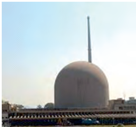
Fig. 5(b): CIRUS Reactor: Outer View of Reactor Building. Fuel details are shown in Fig. 9. (Operations started in 1961)
