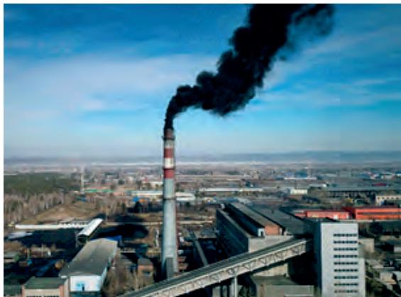
Fig. 2(a): A typical coal fired thermal power station. A typical 500 MWe coal fired unit releases about 10000 tonnes per day of \text{CO}_2 , which has major bearing on green-house effect. In addition, copious amount of \text{SO}_2 , \text{NO}_x gases and harmful Particulate Matter (PM) amongst others are also released. In the year 2021 India emitted about 1.4 billion tonnes of \text{CO}_2 owing to coal firing at power stations alone
