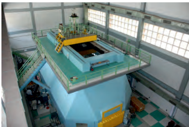
Fig. 6(a): APSARA, the pool type reactor is Asia first reactor which began operations in 1956. The figure above shows perspective view of APSARA reactor along with pool and top bridge houses structures for control rod drives. (see external view in Fig. 5(a))
