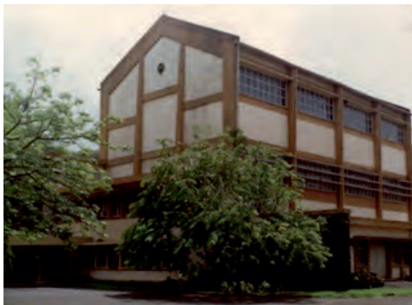
Fig. 5(a): APSARA Reactor: Outer View of Reactor Building. Fuel and Pool Details shown in Fig.6(a) and Fig. 6(b). (Operations started in the year 1956)
