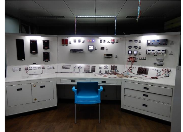
Relay Testing Lab
