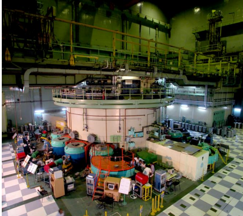
Dhruva Reactor Hall
