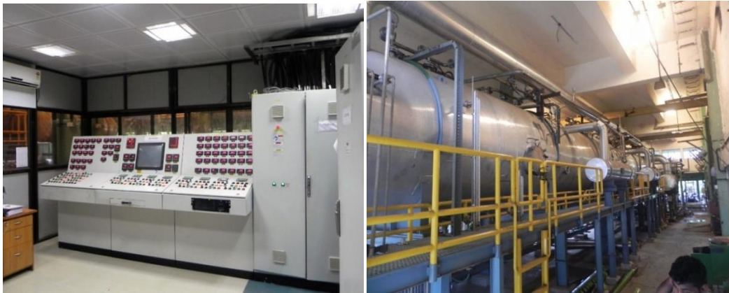
240 m 3 /d capacity MED-TVC plant at BARC
