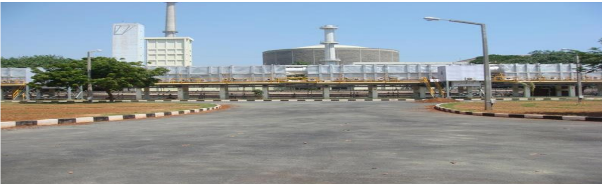
4.5 MLD Multi Stage Flash Plant at Nuclear Desalination Demonstration Plant (NDDP), Kalpakkam coupled to Madras Atomic Power Station
