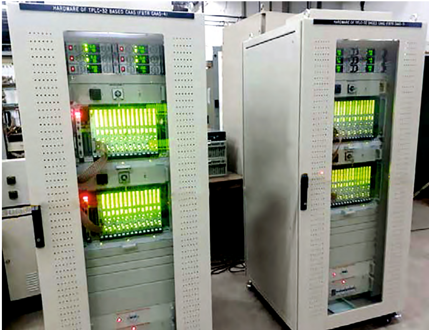
Alarm Annunciation System of FBTR upgraded with TPLC-32 Platform based Computerized System.
