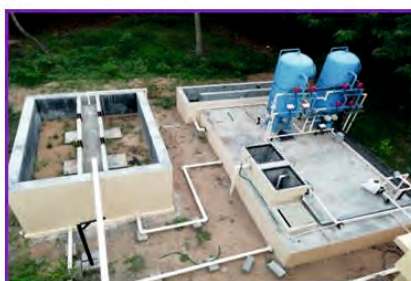
Sewage and treated water sumps, filtration system, drying bed
