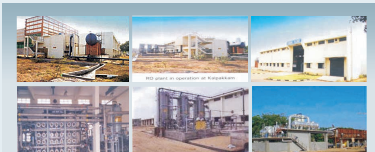
Hybrid RO-MSF Nuclear Desalination Plant at Kalpakkam (6.3 MLD capacity)
