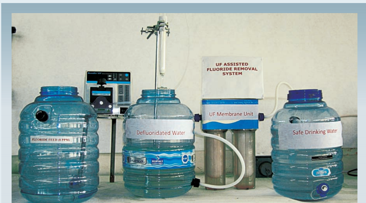
UF Assisted Fluoride Removal System
