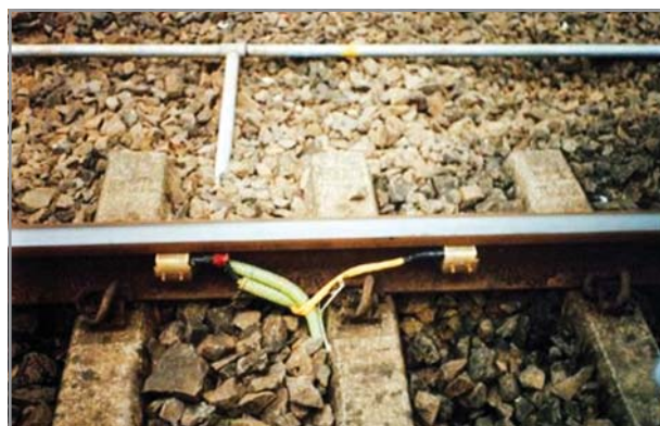
The Train Wheel Detection Sensor installed at Mangoan Station Railway Track of Konkan Railway
